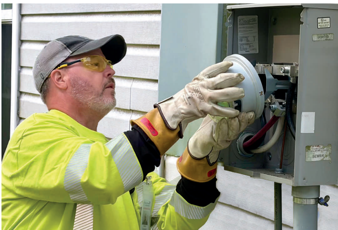
Contractor Steven Glaesman with Border States, a partner of Horry Electric, changes out a 20-plus year-old meter as part of a year-long project to replace aging equipment across HEC's service area.
