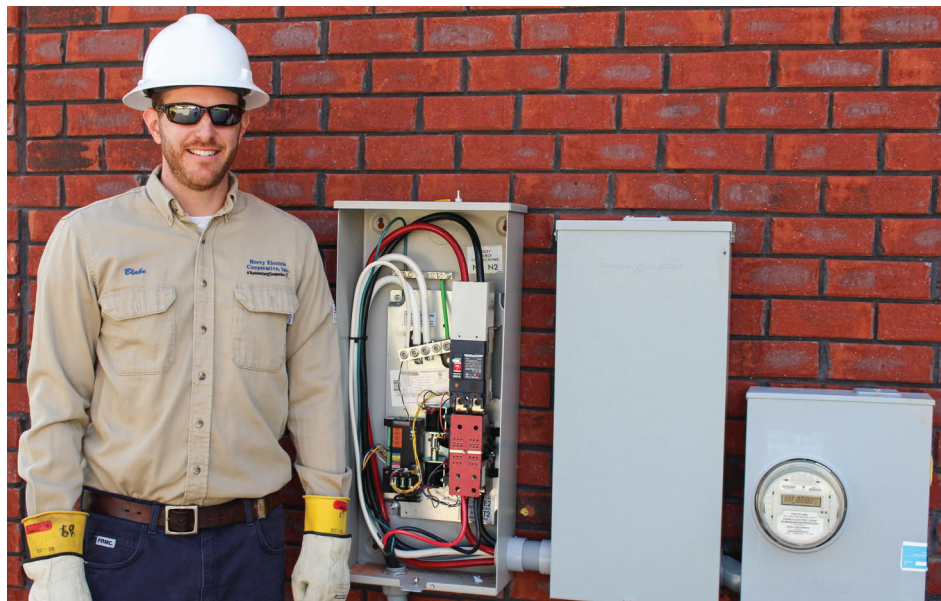
Horry Electric's Metering Supervisor Blake Strong shows the inside of a home generator panel. The panel connects the member's generator to the home circuitry.
