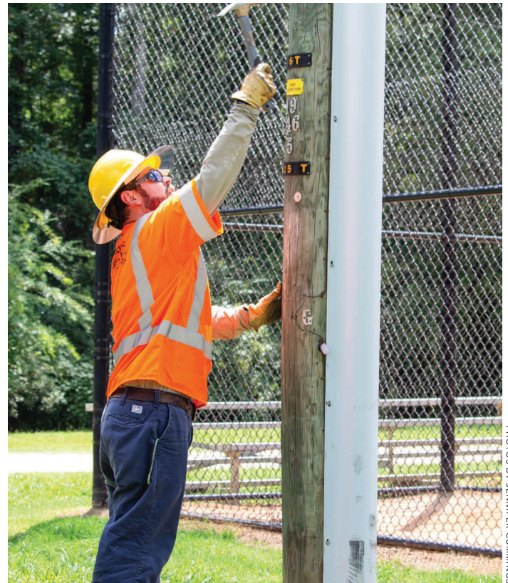
Advanced Line Technician Jacob Riddei checks the condition of a power pole by performing the hammer test. Riddei has to listen for a distinct sound to ensure the pole is not rotting or decaying.
