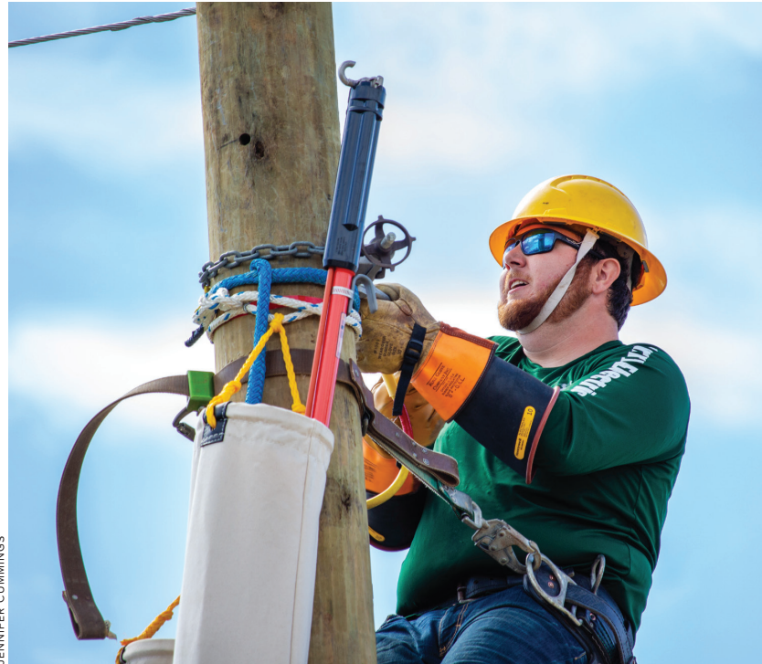
After climbing to the top of a pole, HEC's Jesse Hopkins begins to work on setting up a grounding bracket in the Equipotential Zone Grounding event.
