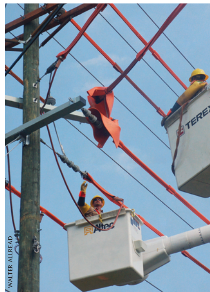
Working on energized lines they've draped with insulated line hoses and blankets, HEC lineworkers Kelly Jordan (left) and Carluss King also use personal protective equipment as they upgrade a "hot" line on Hwy. 544 in the summer heat.
