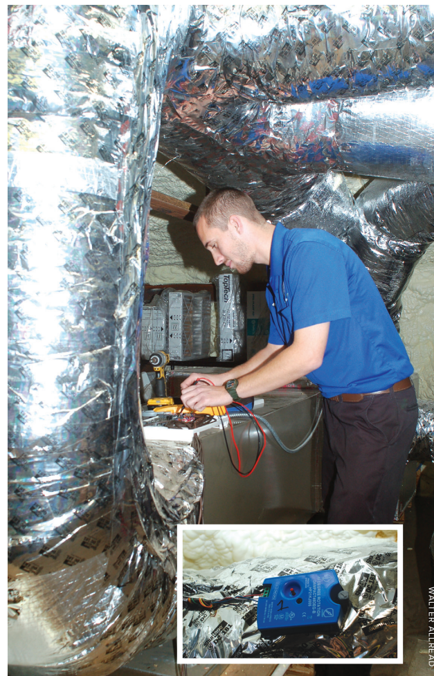
Andrew Seeley, a technician for Conway Air Conditioning, one of HEC's approved contractors, checks a control device for damper actuators (inset) used inside an HVAC ductwork. Dampers control airflow in HVAC systems; actuators are the interface between the control system and the mechanical system. HEC-approved contractors are up on the latest technology and can help you make your home more comfortable and energy efficient. By the way: Seeley is an Horry Electric member at his own home.
