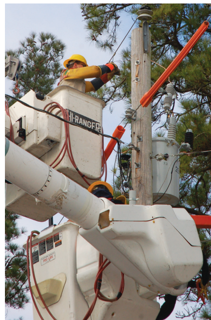
Jeremy Ammons, a first-class lineman for HEC, and Craig Cannon, a B-class lineman, reinsulate a co-op line on Dog Bluff Road. They're using personal protective equipment as well as insulated blankets and line covers to work on an energized line.
