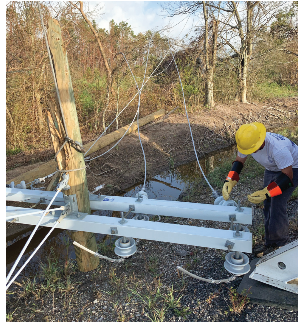
An Horry Electric lineman works on taking material off of a crossarm so crews can begin replacing one of the many broken poles following Hurricane Laura.
